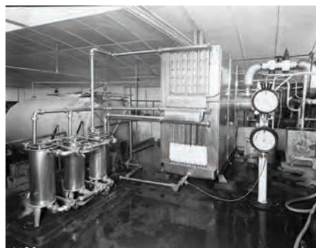
FIGURE 1.22 Pasteurization Equipment
