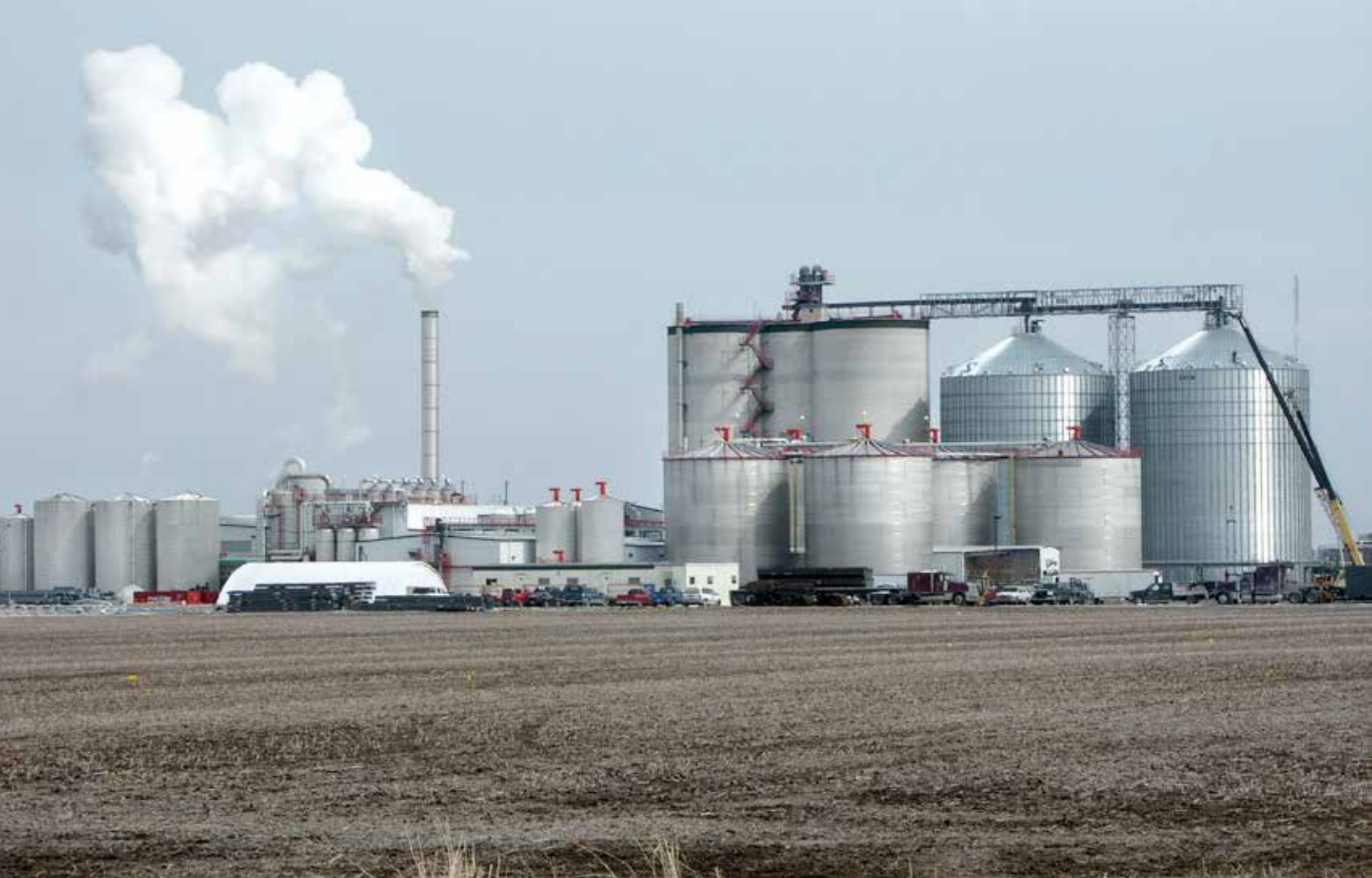
Ethanol plant in West Burlington, Iowa
