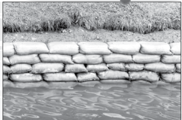
Bags of sand are piled up by the edge of a river. This stops the river water from reaching the riverbank.
