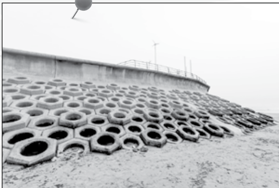
A wall of tires is built on the beach. They help hold the sand in place.
